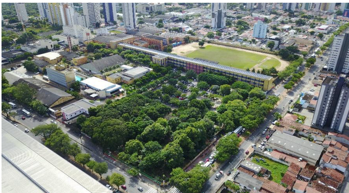
Figura 1 – Vista aérea do IFRN, campus Natal-Central
