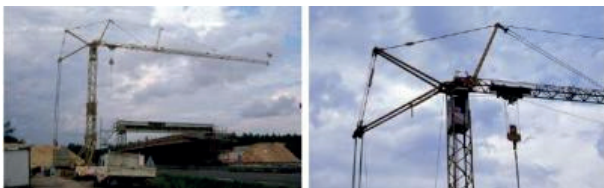
Figure 21. Crane application (Cabo and Bernardo, 2015).
